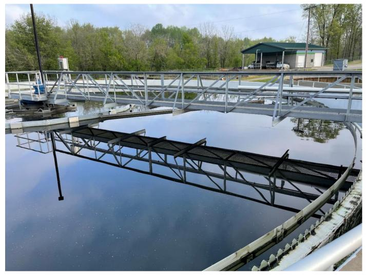
The WWTP has a design biological capacity of 4MGD and a Hydraulic Capacity of Clarifiers around 14 MGD, with extra storage in an Equalization Basin. The plant is operated M-F from 7:00-3:30 and 4 hrs. on the weekend. SCADA is built in with alarms that alert the operators if failure occur.
