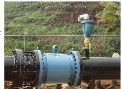
Figure 7. Single Body Combination Air Valve upstream of a Flow Meter
