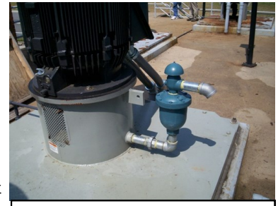
Figure 4. Vertical Turbine Pump with Air/Vacuum Valve
