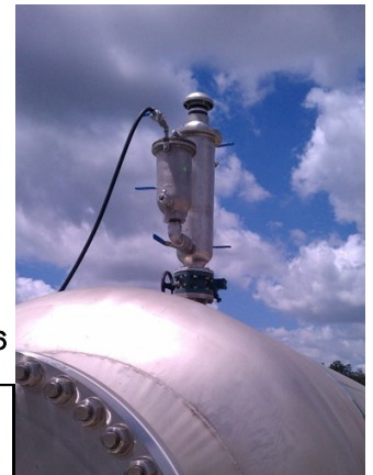
Figure 6. Dual Body, Stainless Steel Combination Air Valve
